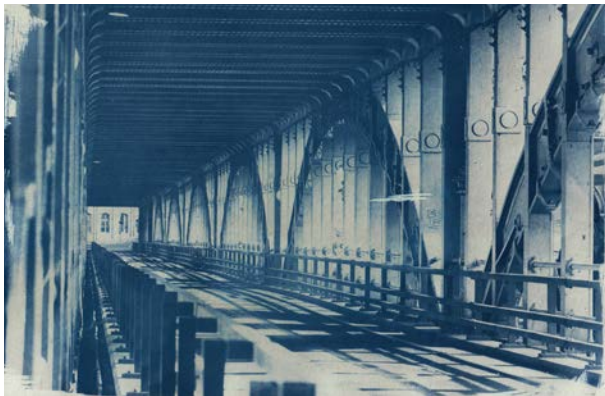
The High Level Bridge , the space between Gateshead and Newcastle, 2024.
