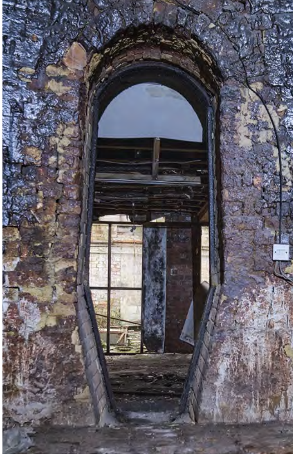
Industry: Bottle kiln, bricks form a heat-proof lining, while the pottery fires., 2022.
